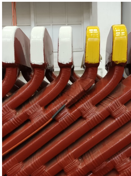
Endwinding vibration sensor on a hydro generator endwinding (IRIS EVAIL)
